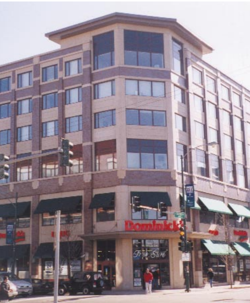
Chicago's first two-story grocery store located at 959 West Fullerton Avenue.
